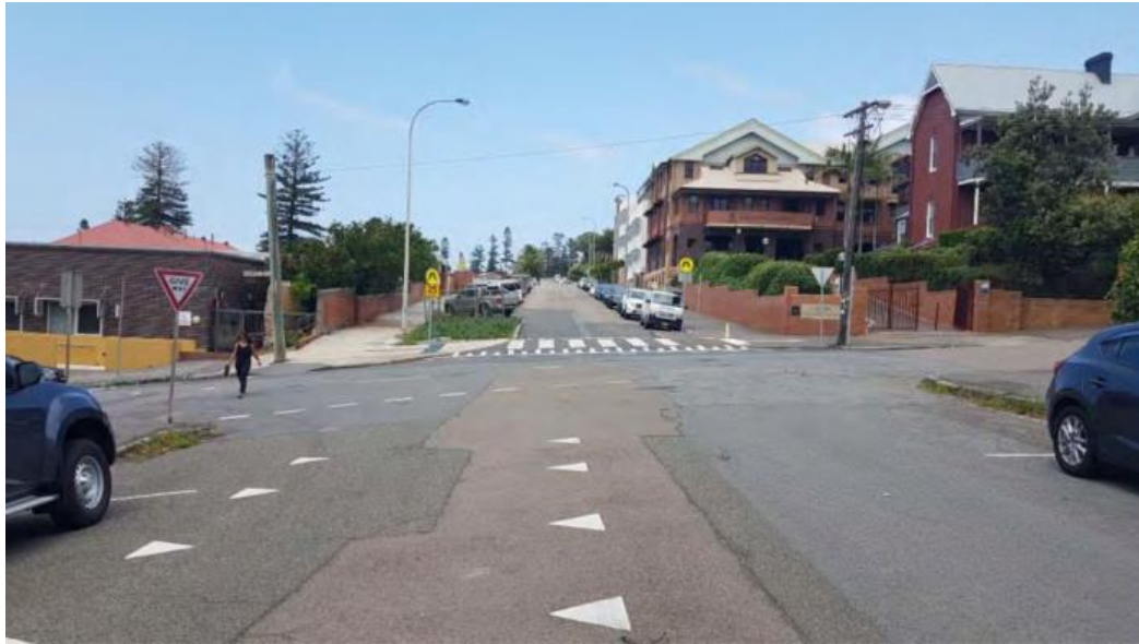
Figure 2.7 – Newcomen Street / Church Street intersection looking South. Note Newcastle Grammar School on the top right.
