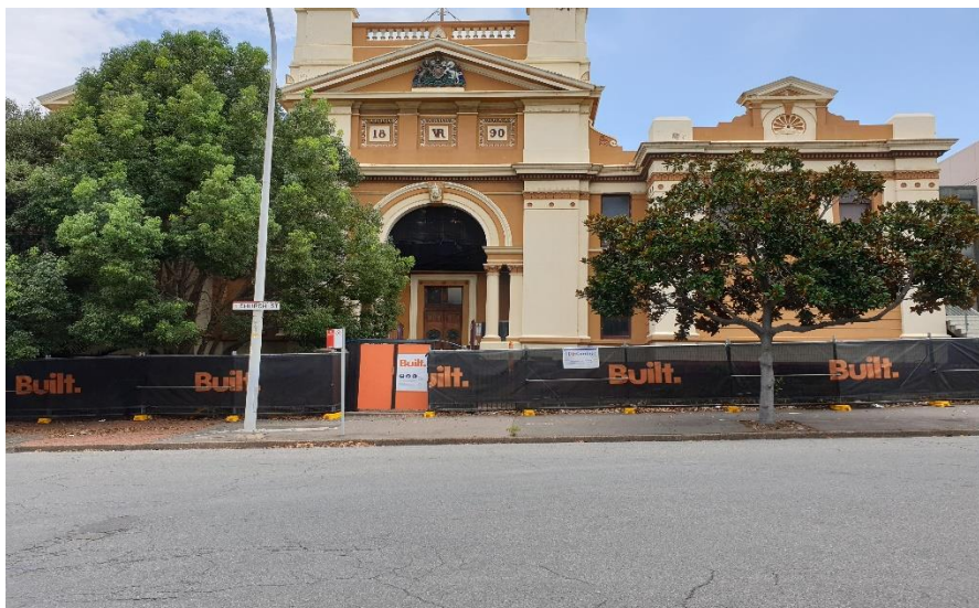
Figure 3.3 – Site personnel gate in orange. Note that this provides safe access directly to site offices and amenities.
