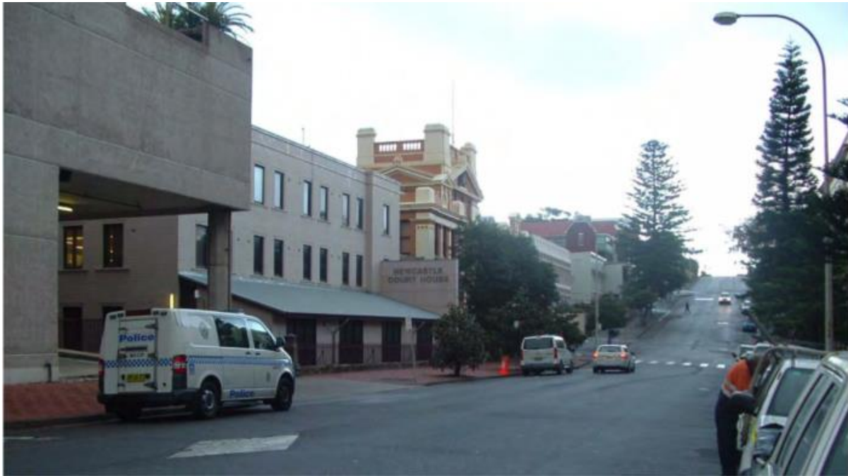
Figure 2.2 - Church Street looking West. Site is on the left with Administration Building in foreground. Note existing pedestrian crossing to be relocated temporarily during works.
